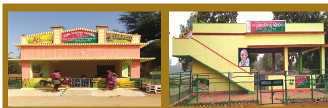
VSS office-cum-Meeting place of Bellahali & Khaliadhipa VSS Bhatlli FMU, Bargarh
