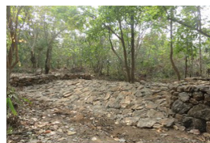
Loose Boulder Check Dam
