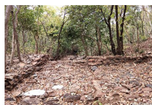
Loose Boulder Check Dam
