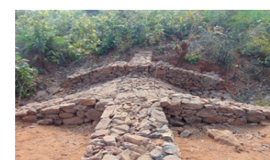
Loose Bounder Check Dam
