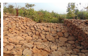
Loose Bounder Check Dam
