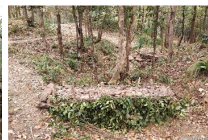
Brush wood Check dam
