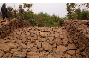
Loose Bounder Check Dam
