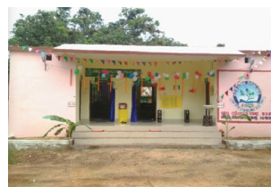
FMU Building, Sadangi, Dhenkanal
