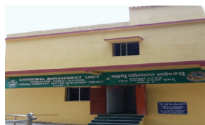
DMU Building, Sambalpur
